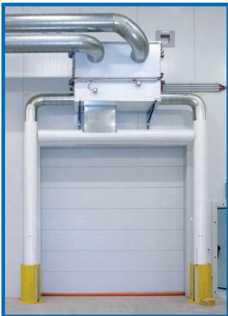
Coldstore logistics doorway
